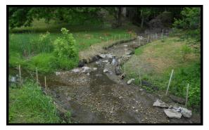
Before this restoration, the tributary had been degraded by road grit, sediment, and trash. It was constrained by a concrete lining and overgrown with numerous invasive species. These unfavorable conditions contributed to the overall poor quality of the stream.
